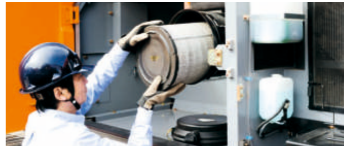
Ground level inspection made easy
